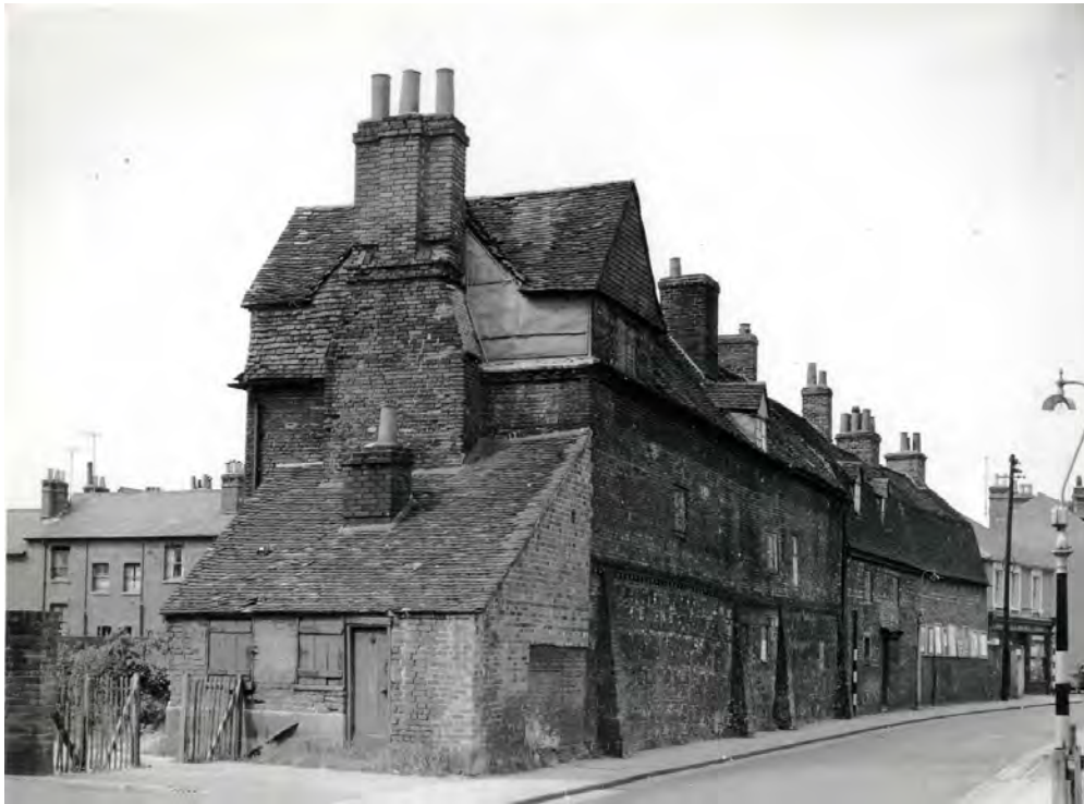
Figure A1.12 Finches Buildings- demolished for the IDR. The side of 3 Baker Street at the far right (source unknown, provided by Alan Stevens)
