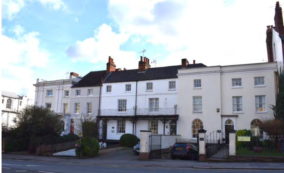
Figure 6.1.14 Attractive diverse terrace of Georgian properties at 113-121 Castle Street (David Neale)
