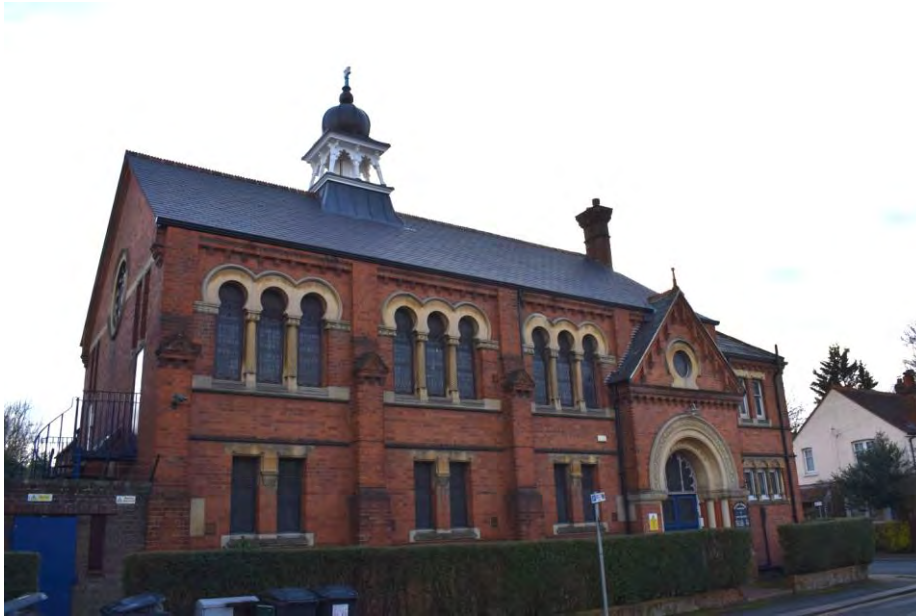
Figure 6.4.9 Listed Moorish style synagogue with fine brick and stone detailing and bell tower, Goldsmid Road at the corner of Clifton Street (Karen Rowland)
