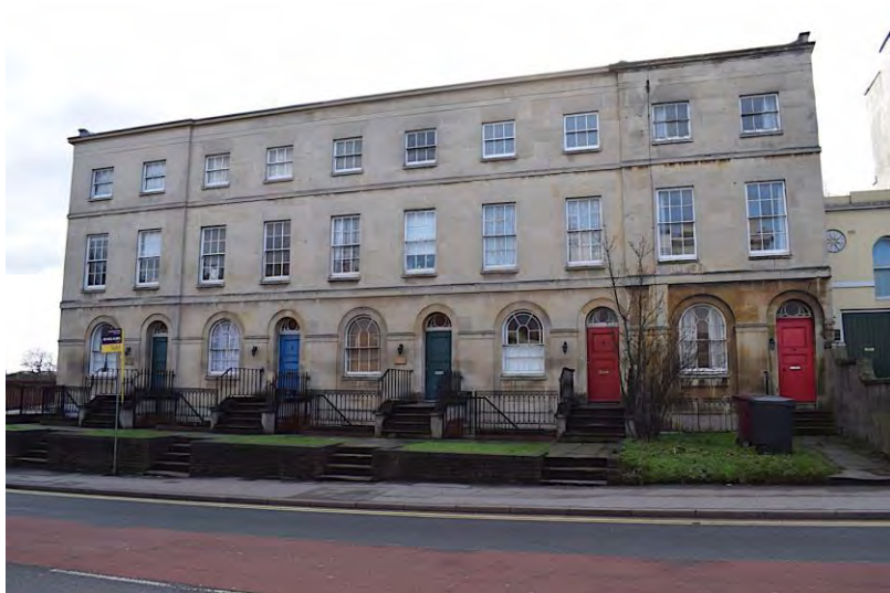
Figure 6.1.12 Blenheim Terrace, Bath stone terrace, 97-105 Castle Street (David Neale)
