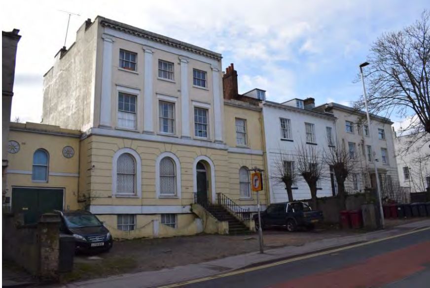
Figure 6.1.10 Large rusticated Georgian houses on the south side of Castle Street at 107-111 (David Neale)
