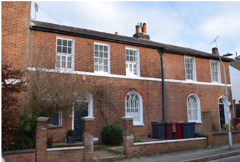
Figure 6.5.4 Arched windows and fanlights on two storey Georgian houses, Coley Hill (David Neale)
