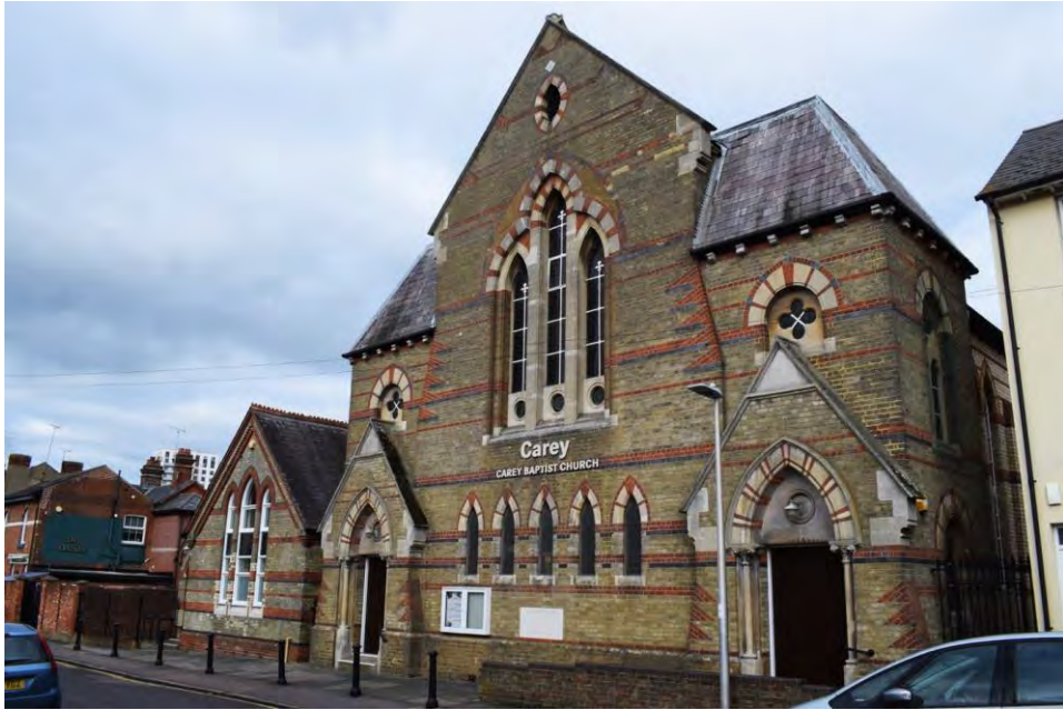
Figure 6.3.20 Carey Baptist Church chapel with its polychrome frontage, 1869 (David Neale)
