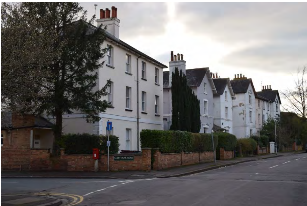
Figure 6.5.6 Stucco 3-storey houses- south side of Castle Crescent near Coley Avenue, c. 1840 (David Neale)
