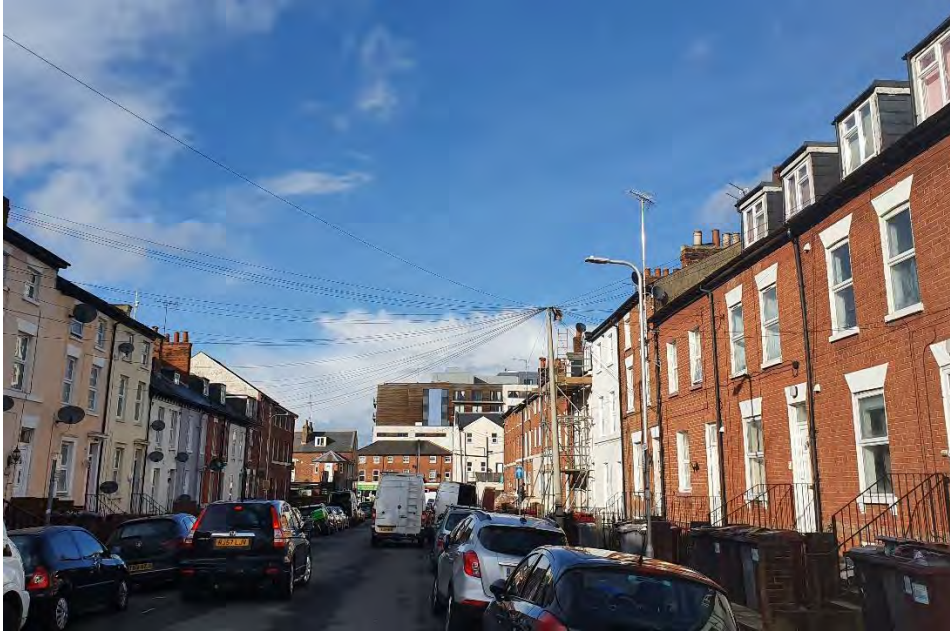
Figure 6.3.17 The conditions of terraced housing looking north along Zinzan Street with poor quality modern dormers, overhead wires, excessive bins and satellite dishes. (Mark Worringham)
