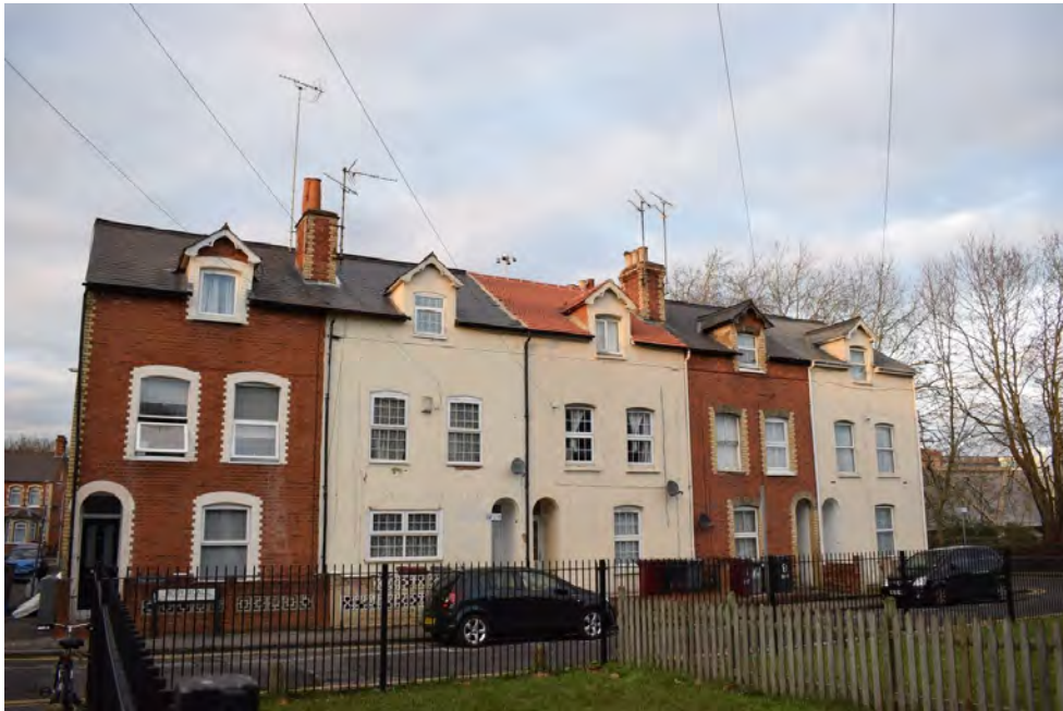
Figure 6.3.21 6-12 Body Road, the new red tile roof was installed in 2017 during the time protection of a conservation area did not apply (David Neale)
