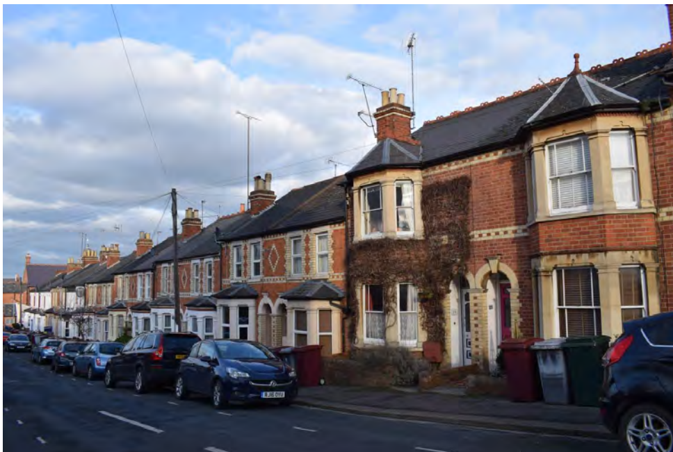
Figure 6.4.7 Terraced polychrome houses along Clifton Street, the ones to the south with double bay fronts (David Neale)
