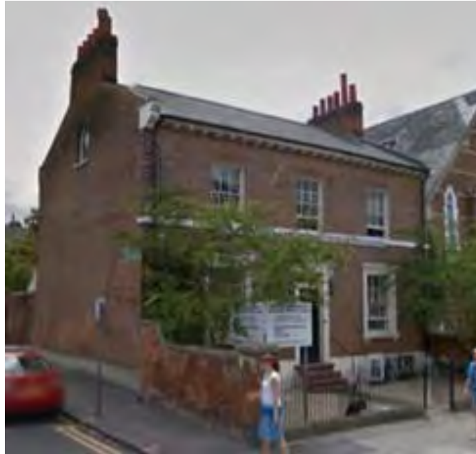
Figure 6.2.5 101 Oxford Road-a detached Georgian family home with original high back garden walls (David Neale)
