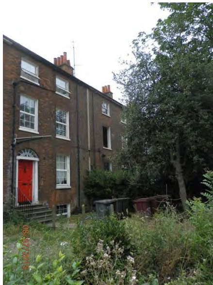
Figure 6.2.8 237 and 239 Oxford Road, part of Prospect Terrace, 237-247 Oxford Road/2 Lorne Street (Reading Borough Council)
