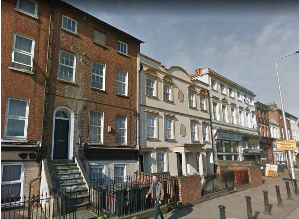
Figure 6.2.3 Oxford Road between Russell Street and Prospect Street - poor condition Georgian terraces, acceptable modern pastiche of pre-existing elements, varied shop façades and poor public realm (Google Maps)
