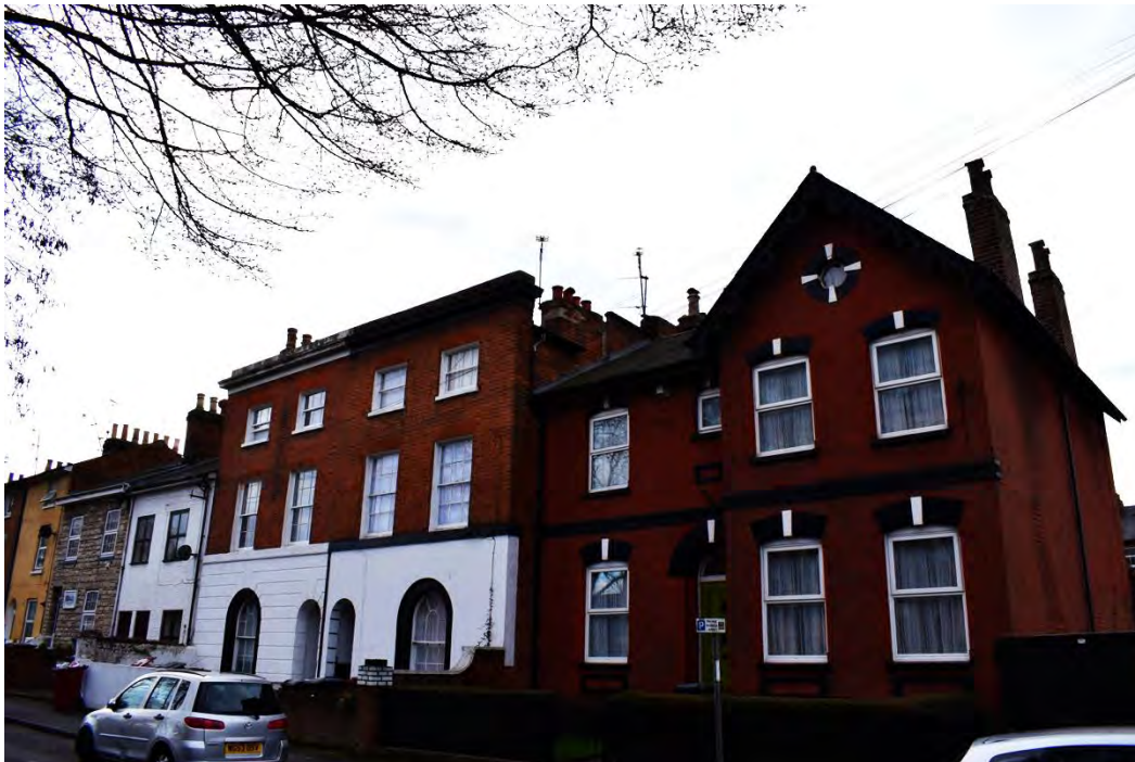
Figure 6.3.4 2, 4 and 4A (listed Georgian semi-detached terrace) Howard Street showing the rustication on 4A (David Neale)
